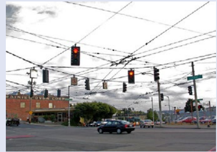
The congestion of overhead utilities in urban street settings poses clearance and driver line-of-sight challenges when traffic signals need modifications for street width and alignment change projects.
