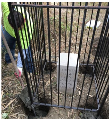
Installation of Fence at SE#8
