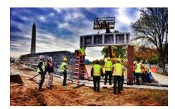
The 17<sup>th</sup> Street Closure is a removable structure that can be erected in the event of high water. It attaches to the floodwalls on both sides of 17th Street and consists of aluminum panels between steel posts. Tis replaced the existing levee, in place since the late 1930s, which consisted of an earthen berm that runs parallel to the Lincoln Memorial
