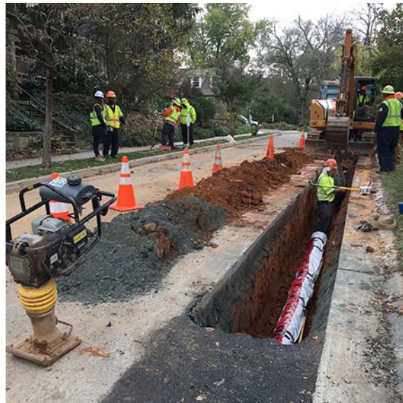
WSSC installing a zinc-coated ductile iron pipe in a trench
