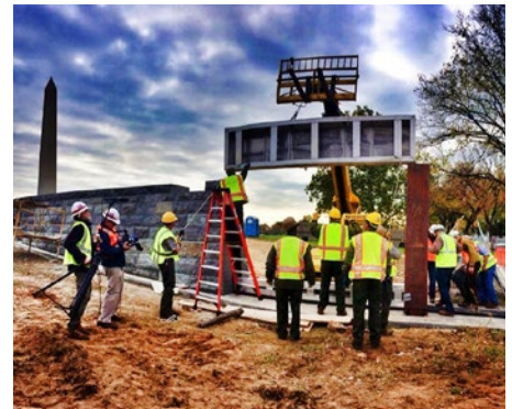
NPS workers practice erection of 17th Street levee
