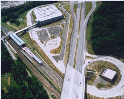
Design on the extension of Metro to Springfield, including the large parking structure
