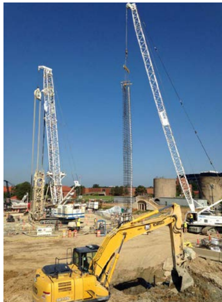
Slurry wall installation south of McMillan Reservoir
