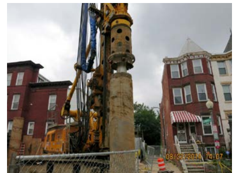
Secant pile drilling at First and V Street NW
