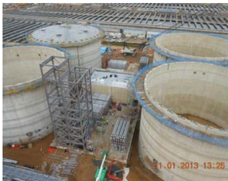
Digesters and Digester Building
