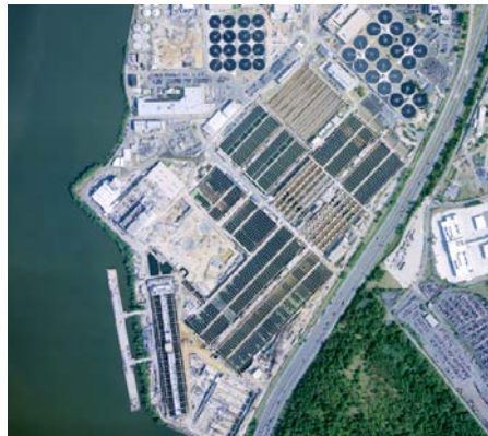
Aerial view of the Blue Plains Advanced Wastewater Treatment Plant
