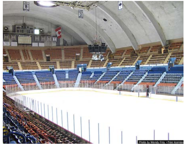
Concrete shell at the Hershey Park Arena.
