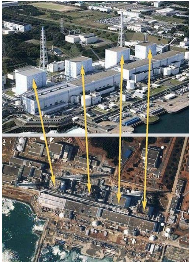
View of Units 1-4 before and after the tsunami and subsequent events at Fukushima Dai-ichi.
