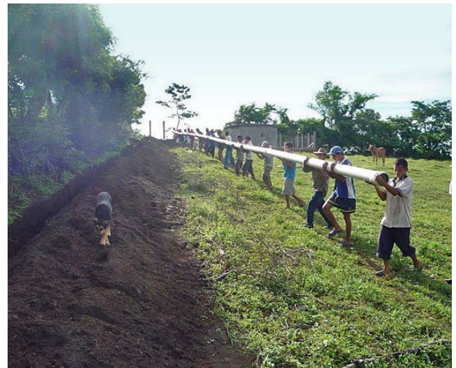
Installing the water pipeline.
