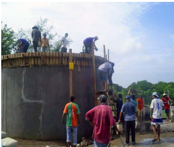
Finishing the water tank.
