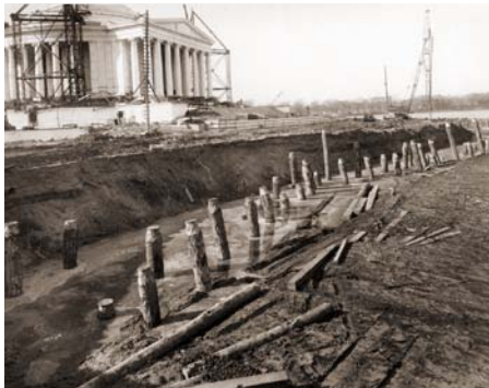
Original Construction – Note timber piles for the seawall.
