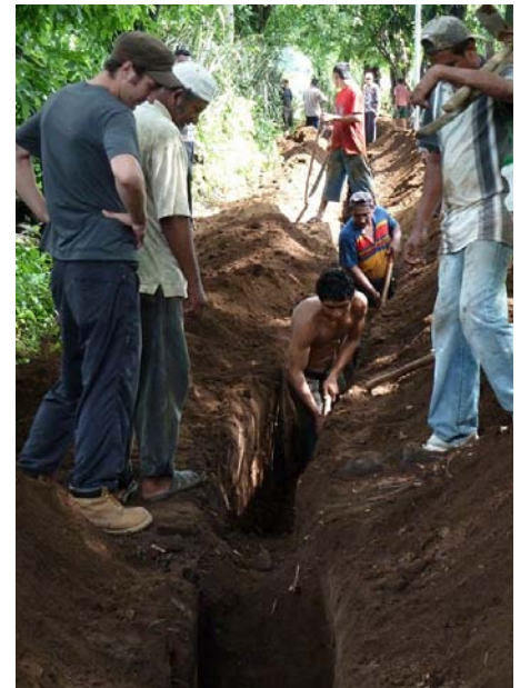
Pipeline trenching the old-fashioned way.
