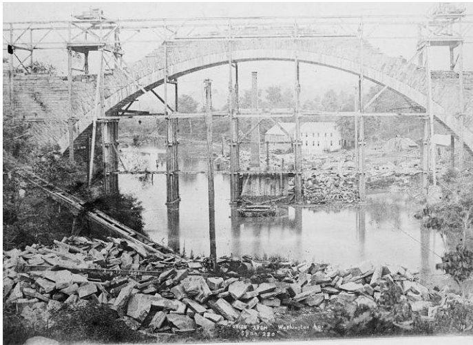
Historic American Engineering Record image – Cabin John Aqueduct Centering Falsework, August 12, 1861
