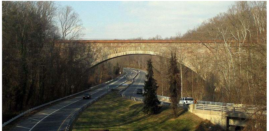
View of Cabin John Aqueduct looking northeast from Clara Barton Parkway bridge.
