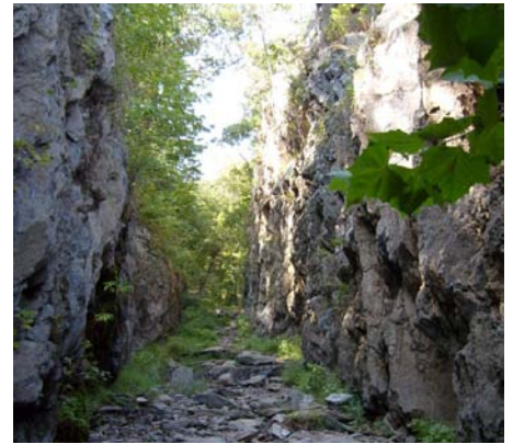
View looking up from Mather Gorge showing the sheer rock walls that were blasted and dug out to construct the lift locks from the river to the upper plateau.
