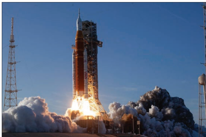
Space Launch System (SLS) vehicle lifting off of the Mobile Launcher—a marvel of civil engineering.
