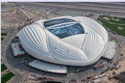
Al Janoub Stadium
