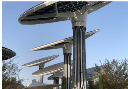
Solar panel collectors within the sustainability district
