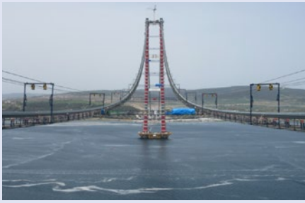
Main cables of Cannakale 1915 Bridge, Courtesy of COWI A/S Denmark
