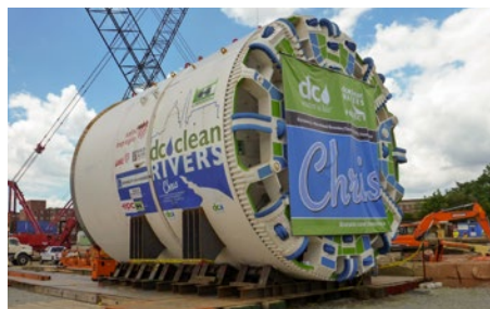
"Chris" the TBM
