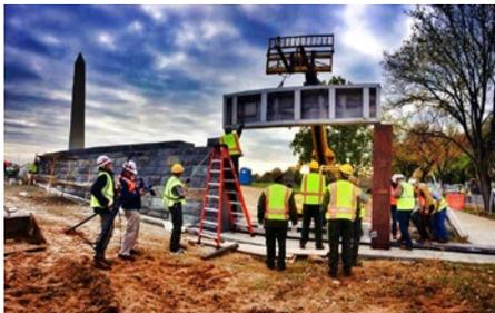
The 17th Street Closure is a removable structure that can be erected in the event of high water. It attaches to the floodwalls on both sides of 17th Street and consists of aluminum panels between steel posts. It replaced the existing levee, in place since the late 1930s, which consisted of an earthen berm that runs parallel to the Lincoln Memorial
