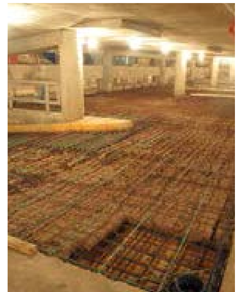
Prepared Repair Area With Steel Replacements
