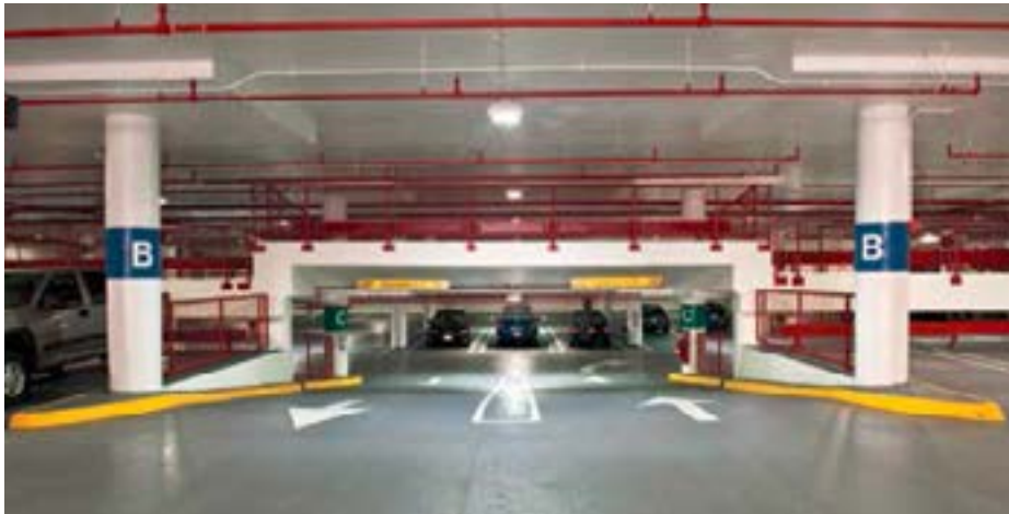
Completed Parking Garage Interior
